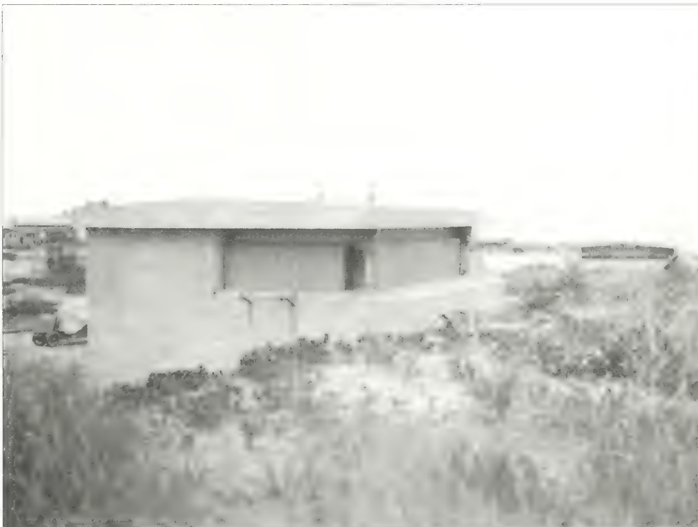
Figure 2.82. Covered battery commander's station at Battery Peck, 1921. In concert with the alterations made at Battery Engle, a fully-enclosed, concrete, battery commander's station, center, was added at Battery Peck. The coincidence range finding station constructed on top of Battery Engle can be seen on the right (Thomas Hoffman, Fort Hancock , Charleston, SC: Arcadia Publishing, 2007).
